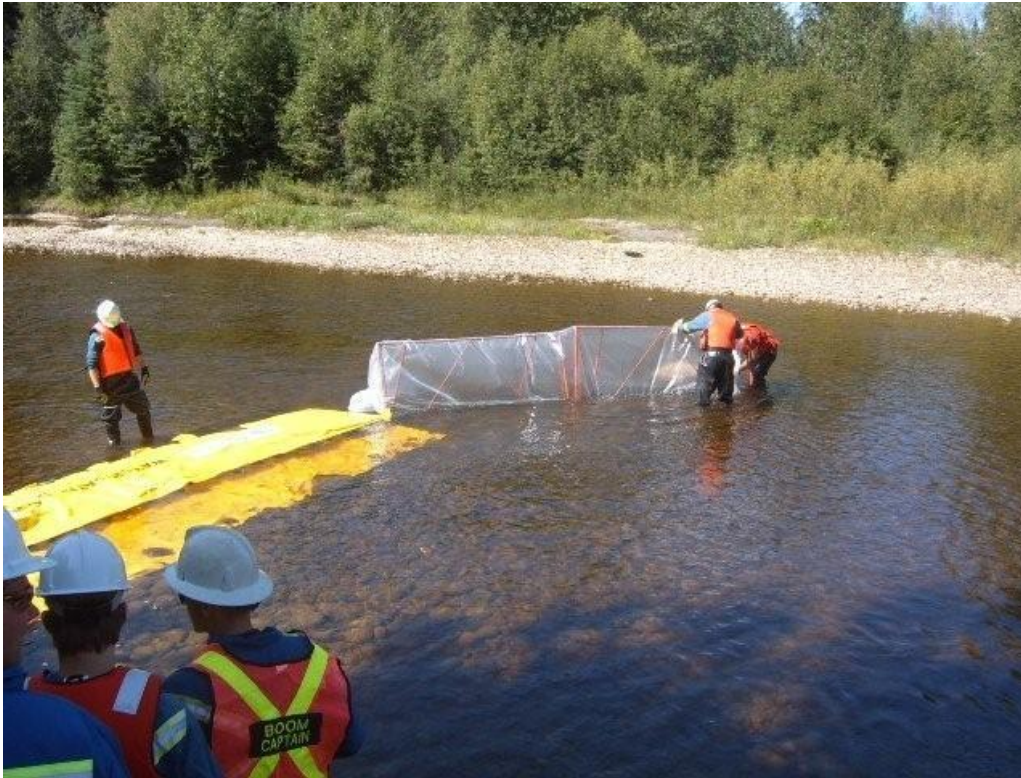
Watergate Dam & Turner Valley Gate – Area W 2010 Exercise
